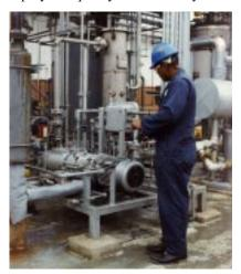
At Allied Colloids, use of the COBRA C400 has been a success. In addition to generating vacuum levels need to maintain polymer integrity, this environmentally friendly.
